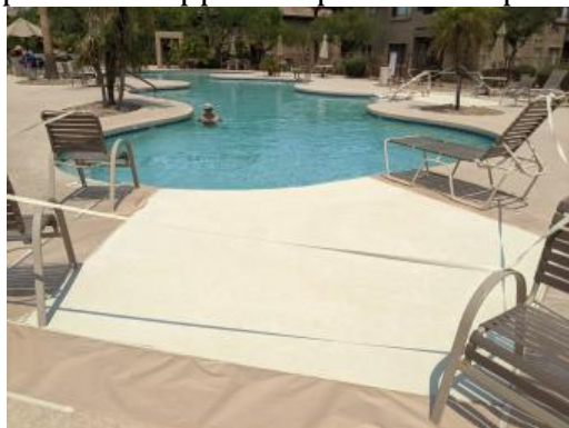
Poolman repairing pool deck
