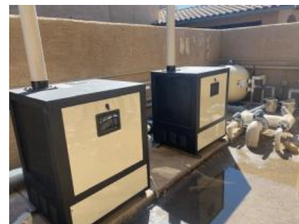
Two new pool heaters
