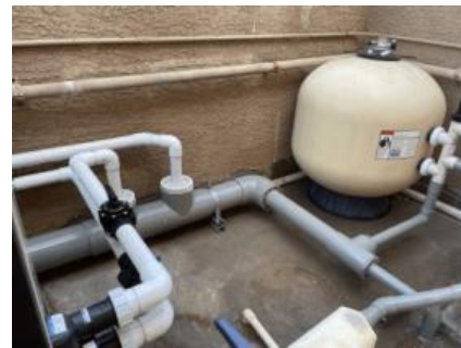
Pool heater mandated new plumbing
