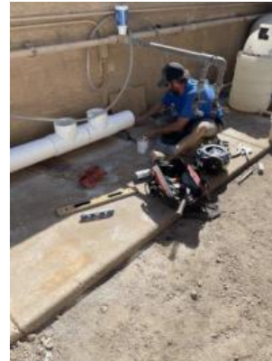
AAA Technician installing new heater plumbing
